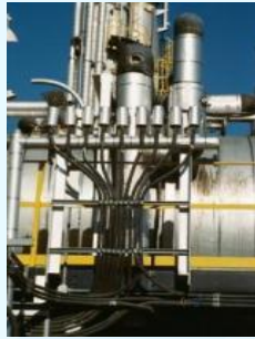
Transport Processing Distribution
